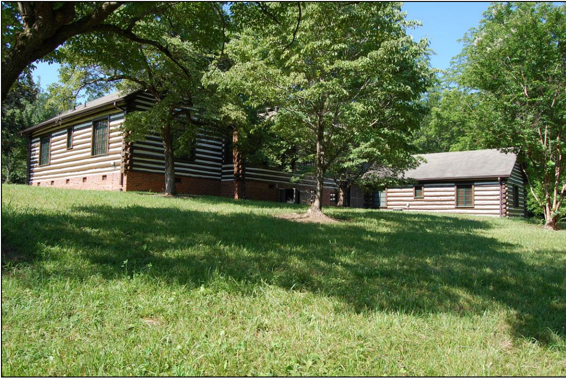
Figure 15. North rear and east side elevations of Morgan house
