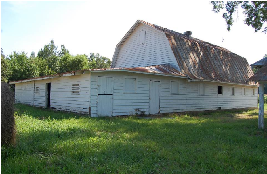
Figure 19. Enclosed stalls wrapped around long south and west gambrel-end of stable
