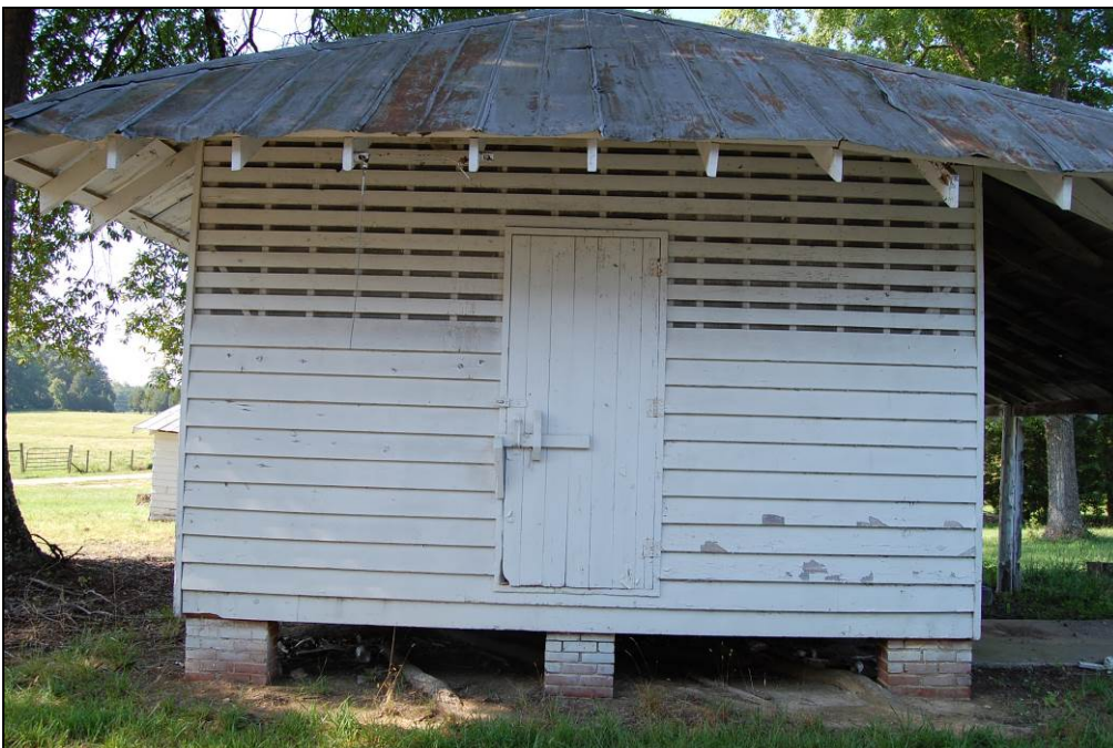
Figure 22. North elevation of corncrib
