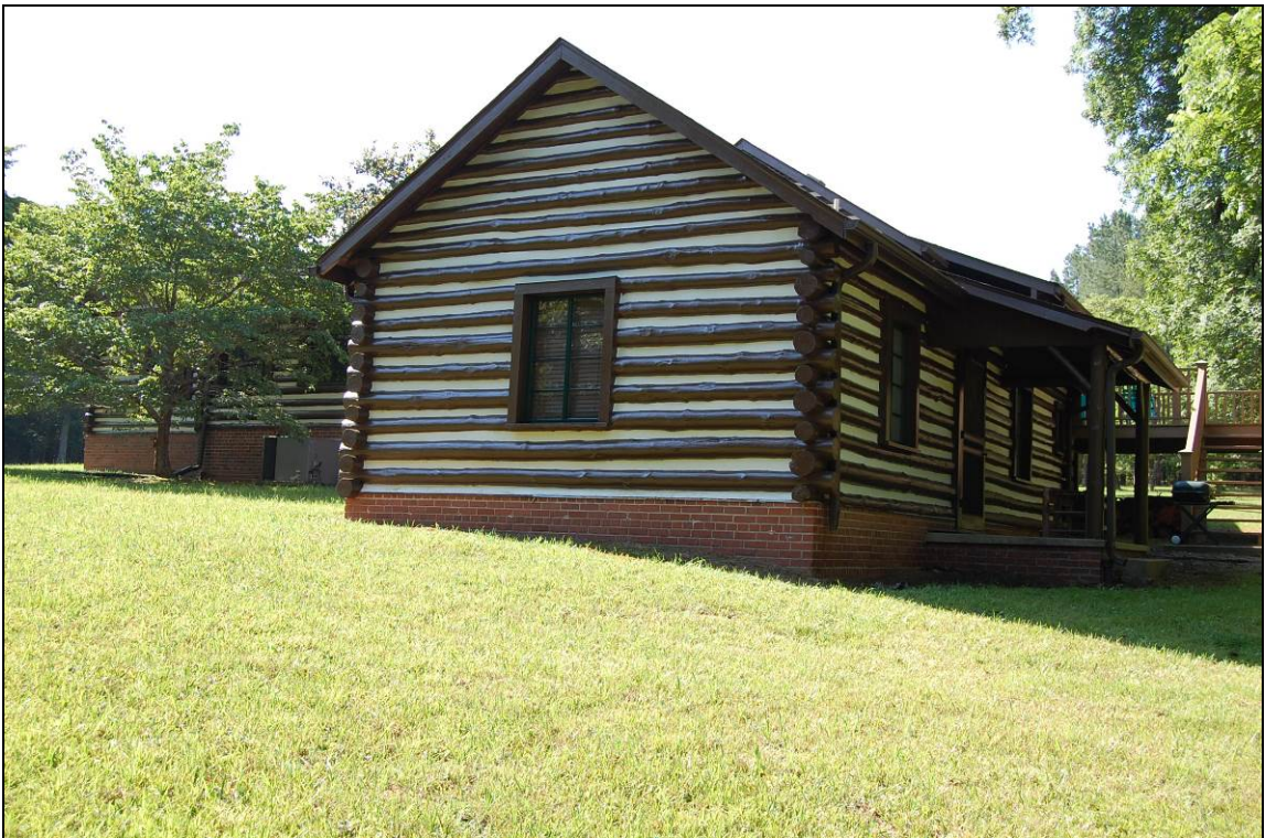
Figure 14. West side and north rear elevations of Morgan house and ell
