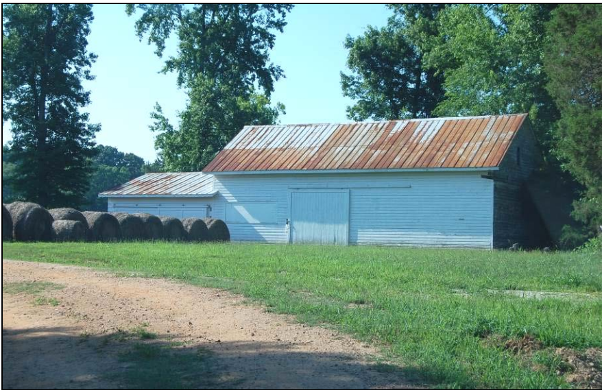
Figure 17. Long north and west gable-end elevations of pack barn with original block at right
