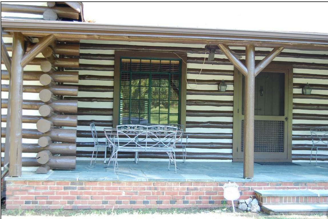
Figure 12. Front porch of Morgan house with log posts and upbraces and fixed and casement window
