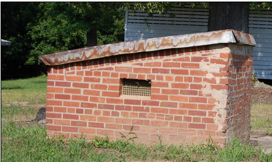
Figure 28. Looking northwest at pumphouse with corncrib to rear
