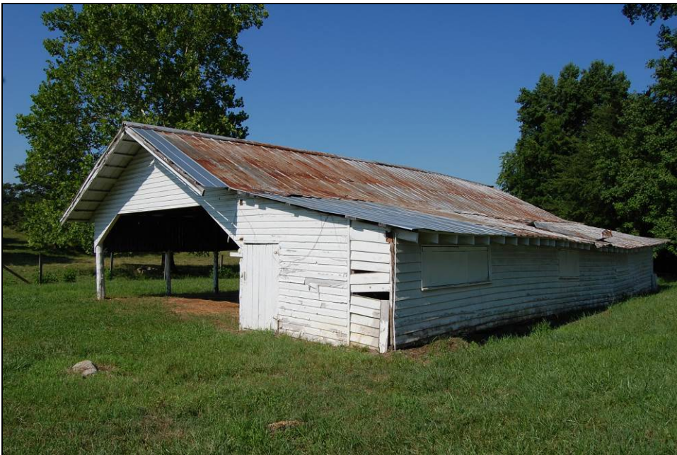
Figure 26. Long north and gable-end east elevations of equipment shed
