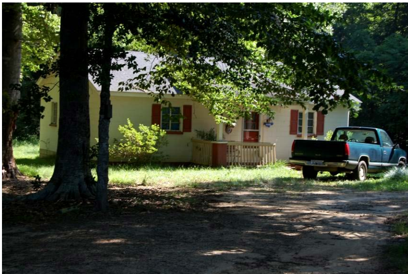
Figure 35. West side and south front elevations of tenant house
