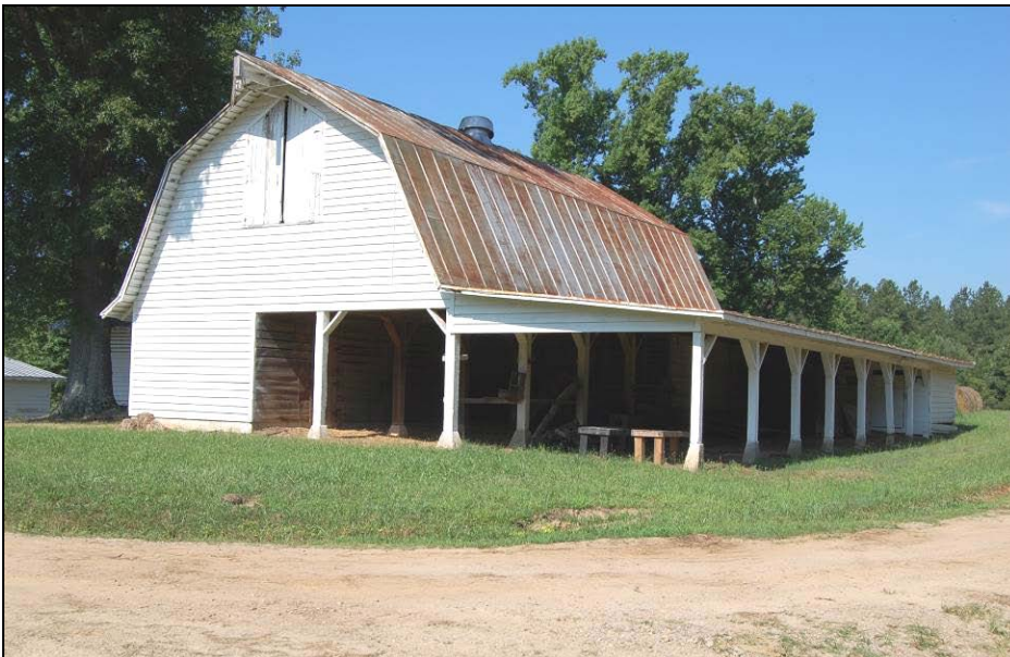
Figure 20. Open shed along long north elevation of stable at notched-in northeast corner of building
